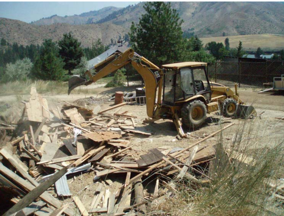
Demolition of old fire barn underway.
